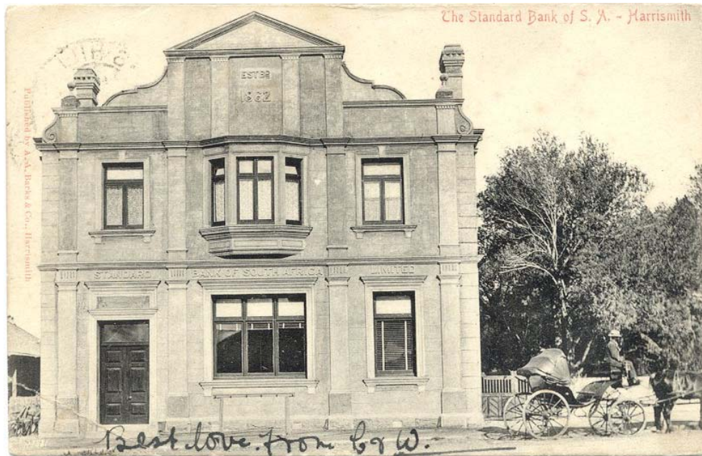
The Standard Bank of South Africa Harrismith
